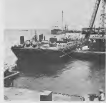
AFTER SLIPPING into the water via the marine railway, the barge was secured for touch-up operations. DESPITES D slip den awa via e marine railway, e barge a wordé mará pa toques final.
